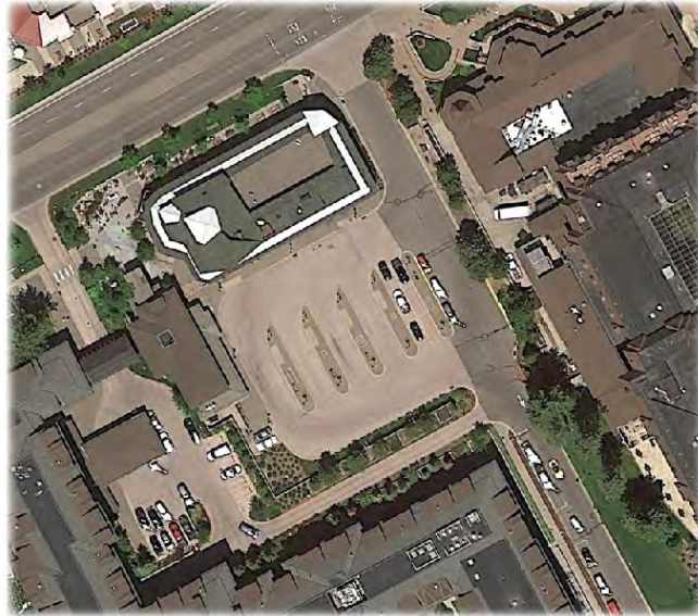
Figure 6-3 - Stateline Transit Center
