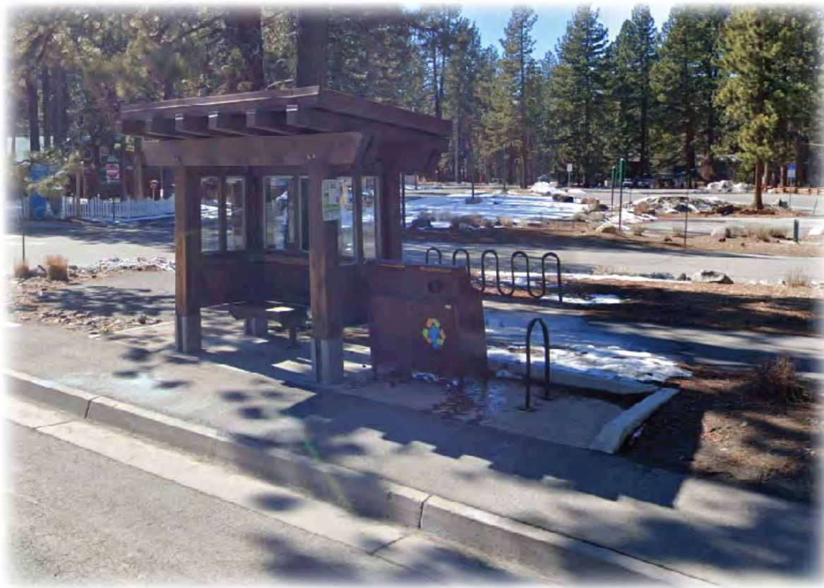
Figure 6-9 - Bus Shelter with Bike Racks
